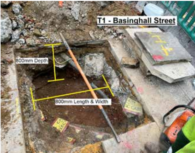
Trial hole excavation
